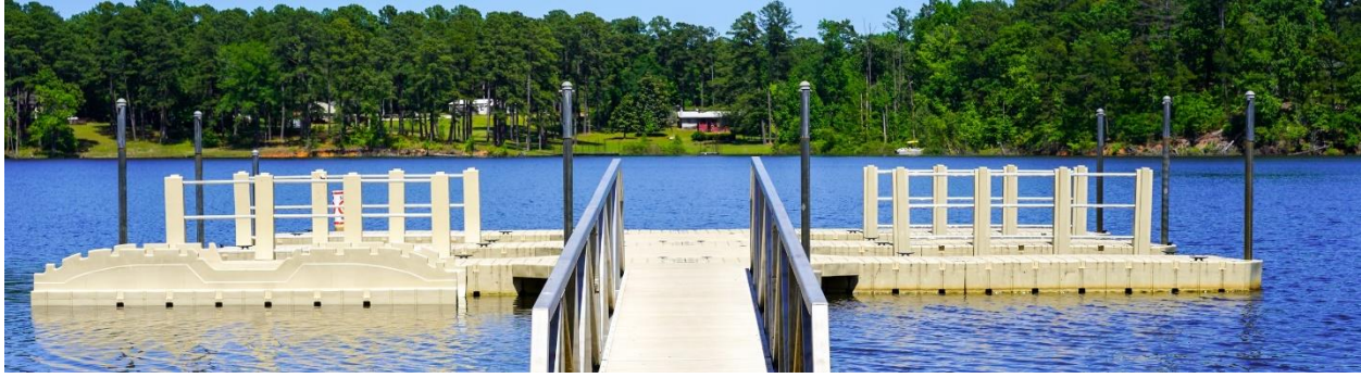
Johnson Creek courtesy dock with added safety handrail and kayak/canoe launch.
